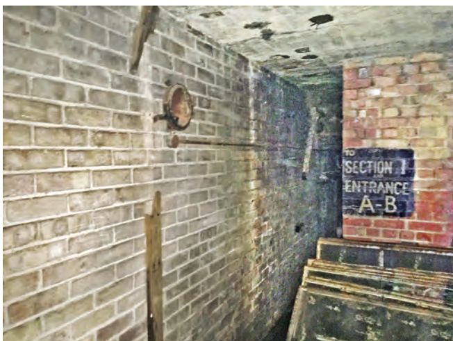
The brick-lined tunnel remains in good condition. Photo Ian Walker
